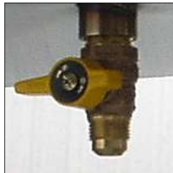
Figure 4b, drain valve enlarged to show detail
